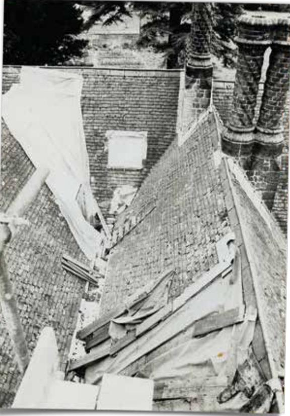
*The roof of Chitfurst House was designed in 1861 to collect rainwater which was channelled down through the house to an underground well.*
